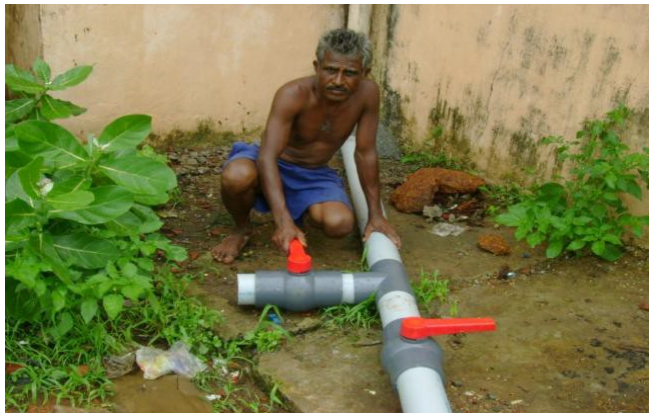
Fig. 2: Foul Flush Mechanism to divert first rains
