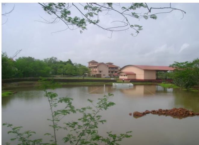
Fig.6: Synoptic view of the rainwater harvesting Lake
