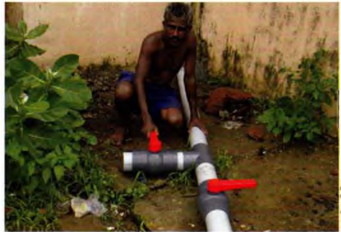
First flush device in use in the roof top RWH site on campus
