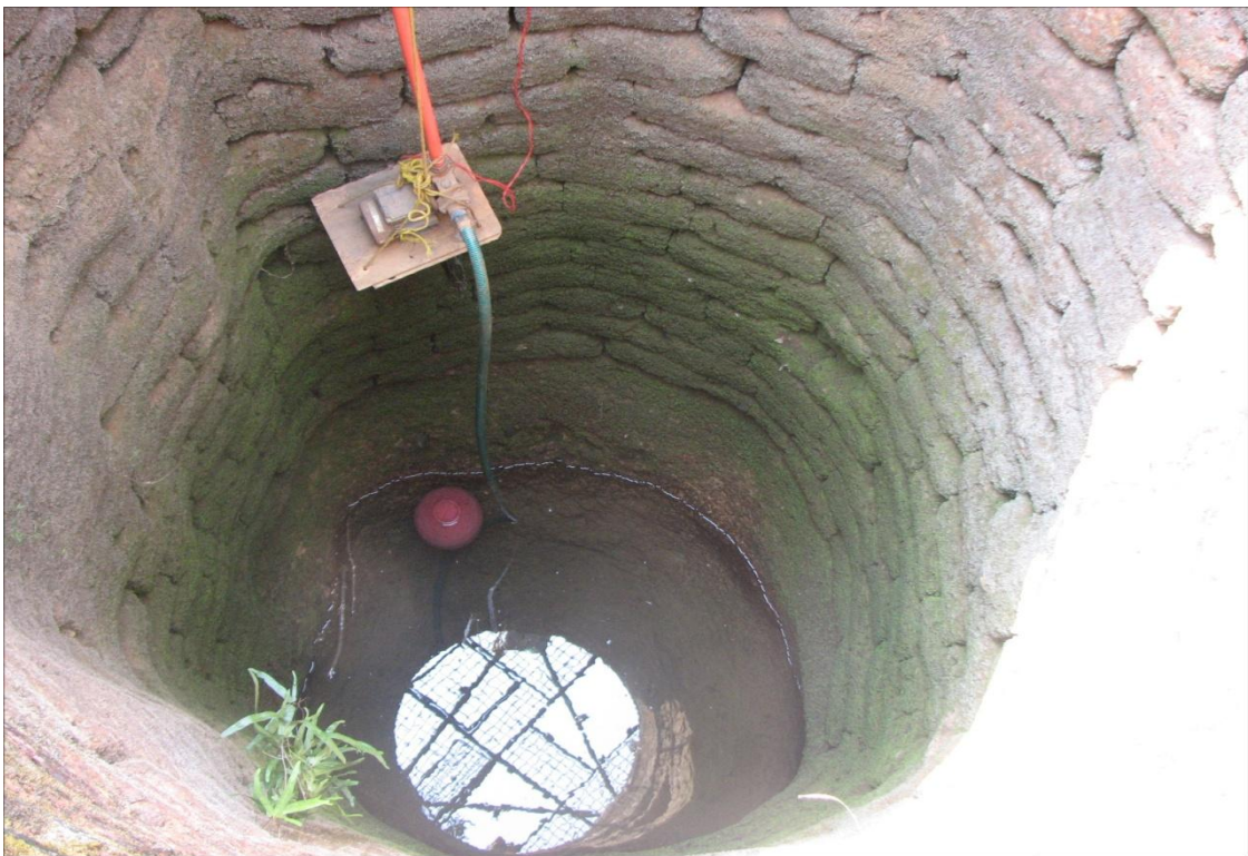
Plate 4.1 A section of laterite weathering profile developed upon the metamorphic rocks (upper photo) in the Mhadei River watershed and a typical circular dug well in laterite (lower photo). Note the protection wall constructed to avoid caving in of loose laterite.
