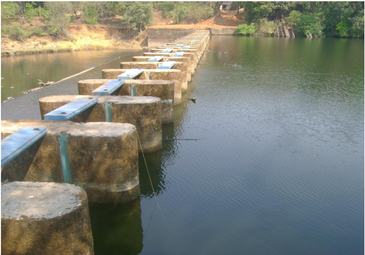
Plate 5.1 Pictures of bandharas built across the Mhadei River channel at Sonal and Ganje
