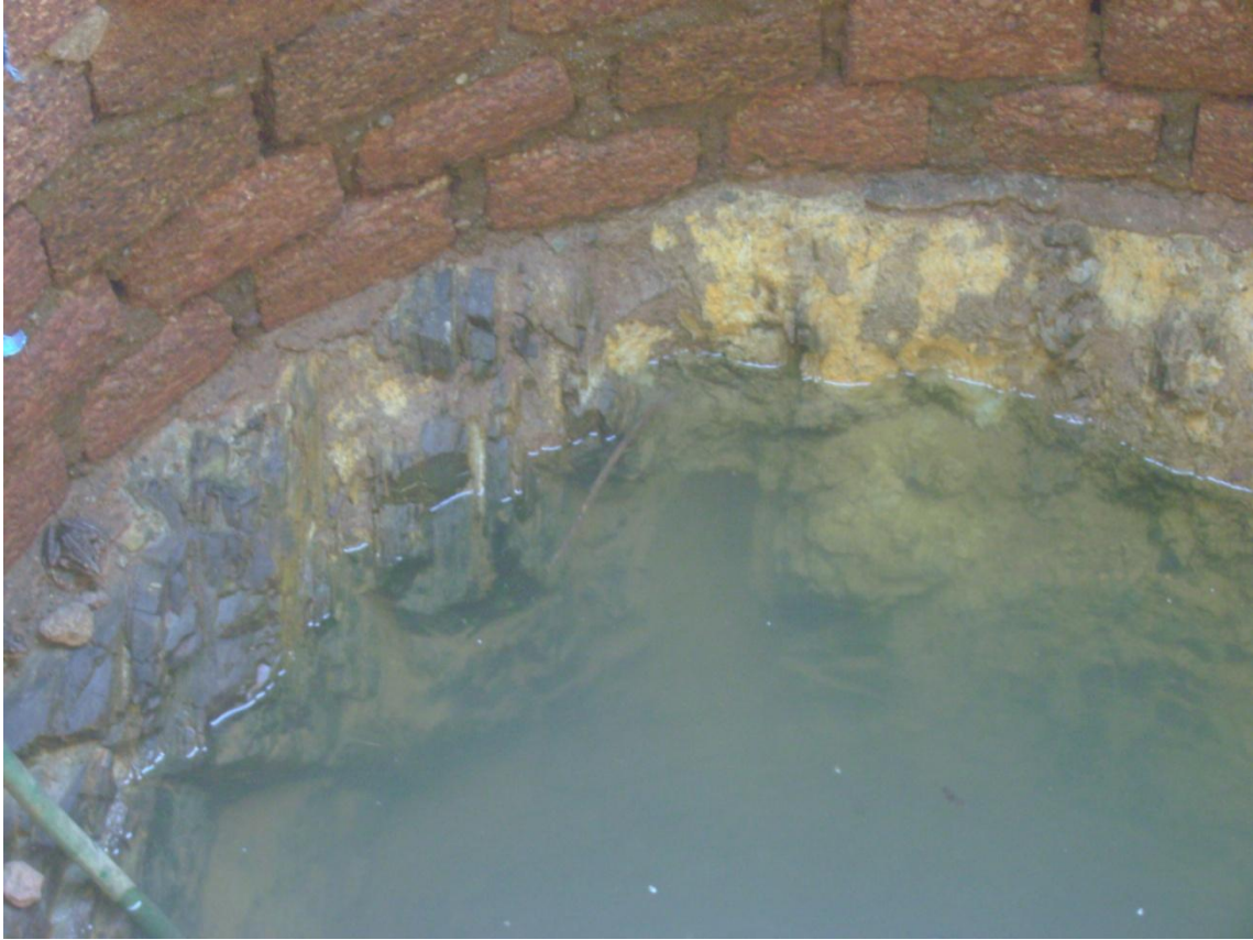
Plate 4.4 Photograph showing an open dug well tapping the semi-confined aquifer in the fractured and weathered schistose rocks in the Mhadei River watershed.
