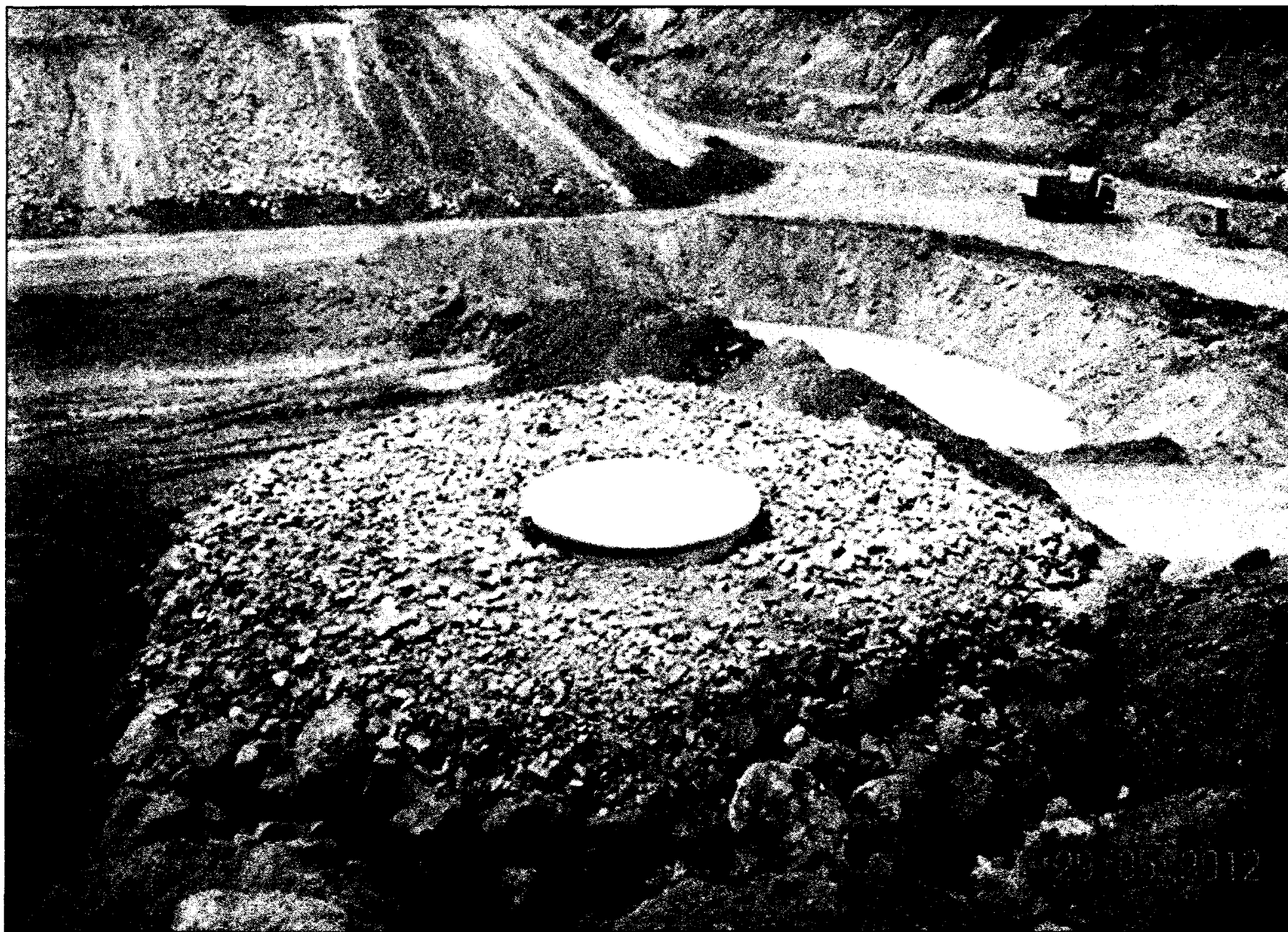
Fig. 7:Well covered with metal cap for safety
