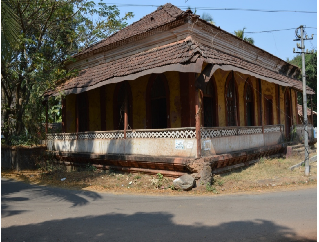
Photo 7.1: An Empty dilapidated house in Bencleamvaddo, Cuncolim
