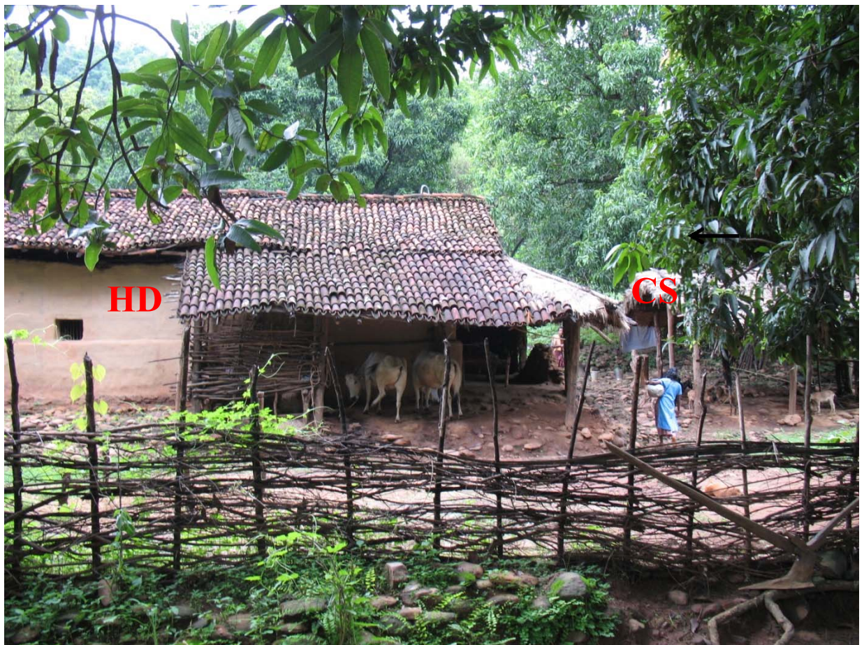
Figure 2: Household having mud plastered walls and tiled roof with adjacent cattle shed in HF ecotype
