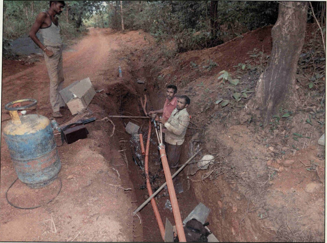
Photo 6.1: Underground cabling done in tribal hamlets
