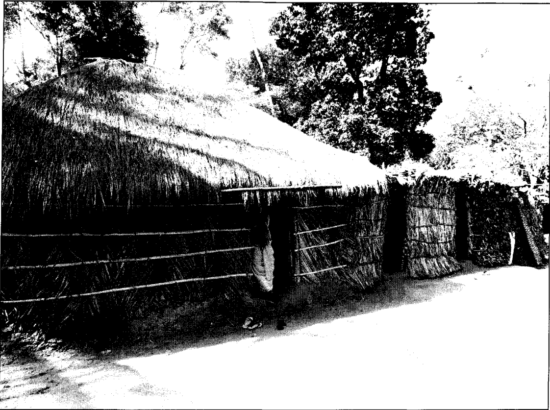
Photo 4.4: Temporary houses at Daando
