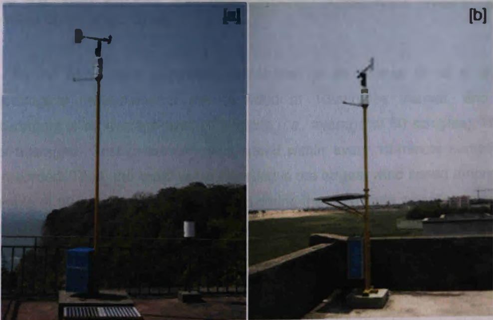
Figure 2.8. A typical installation of AWS in NIO's ICON at [a] Ratnagiri, Maharashtra and [b] Gopalpur, Odisha.
