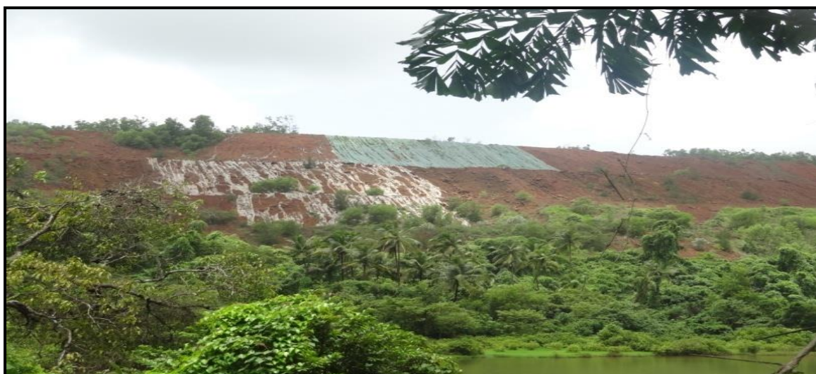
Fig 4.1.1.c Photograph showing mining dumps that have been kept unprotected and unstabilized on the bank of Bicholim River (BR), Goa-West coast of India
