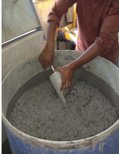
(a) Mixing of concrete
