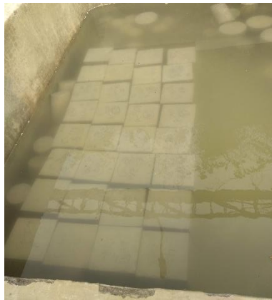
(c) Curing of concrete cubes
