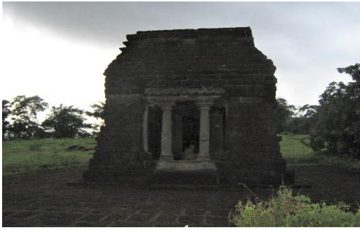
Figure 3.1: Mahadev Temple of Angod Curdi, dismantled and reconstructed by ASI at Salaulim.
