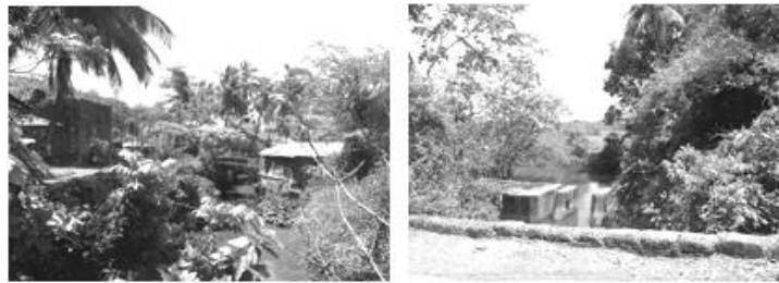
Figure A15.13 Old Lateritic Stone Arch Bridge Culvert and (b) ancient sluice gate on Tembi Rivulet.
