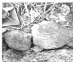
Figure A15.37 Reinforce with rice straw, and compact with 25 blows of 10 kg hand-rammer
