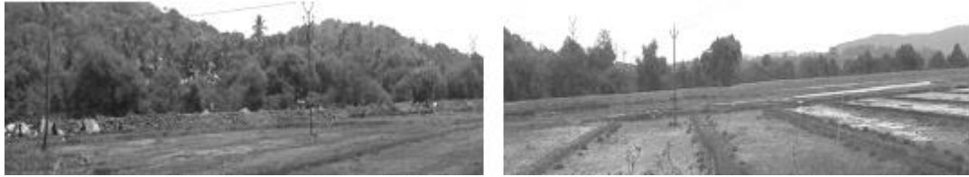
Figure A15.16 Damage and flooding immediately during construction itself
