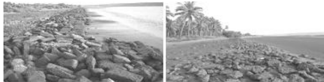
Figure A15.4 The Quay Wall with the start of the breakwater and the destroyed TGSB
