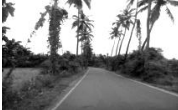
Figure 1.8 Transportation Infrastructure: Road on TGSB
