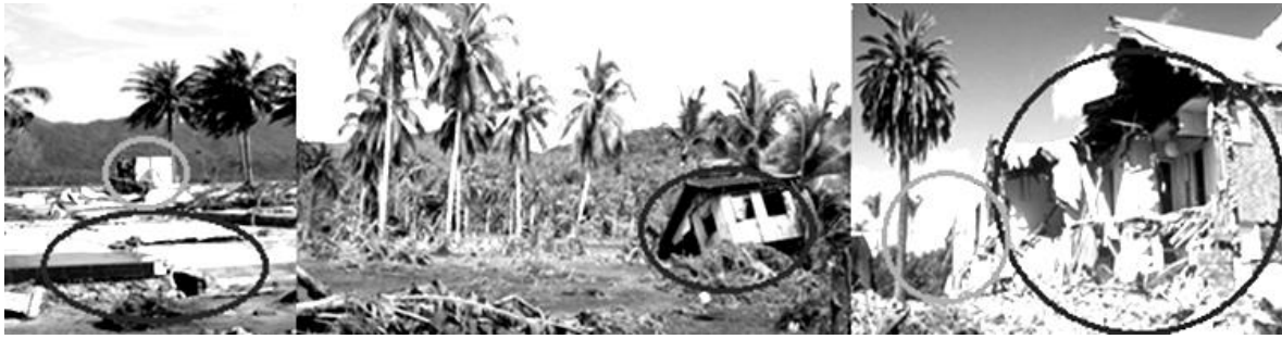
Figure 3.23 Random internet photos show structures nearer palm trees suffering less damage while structures away show more damage.
