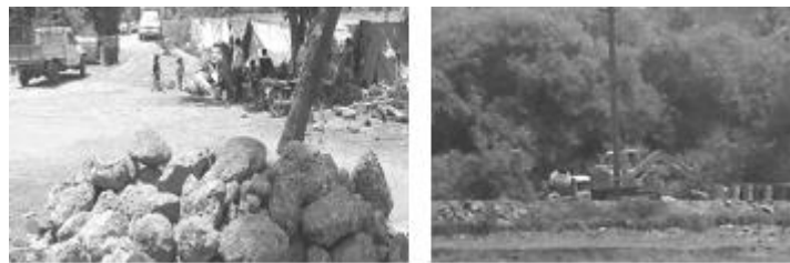
Figure A15.14 Untrained labour(no masons) and equipment used for construction
