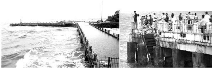
Figure A10.4 (a) Donna Paula jetty inundated by huge waves as cyclone approaches (ToI) as a 2 m storm surge makes the water touch the top of the jetty.
