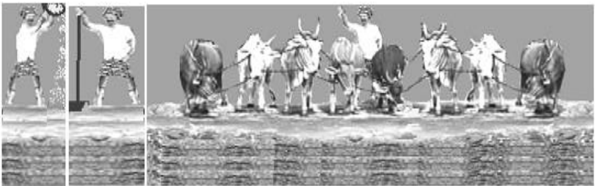
Figure 3.6 Compaction of TGSB by tamping and bullock chain
