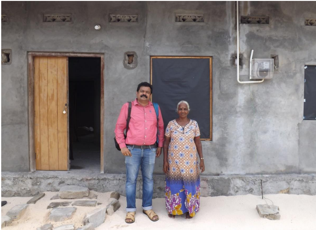
Photo 2: It was routinely observed during fieldwork that owing to unplanned construction, many houses were left unfinished after plastering, with families living in them
