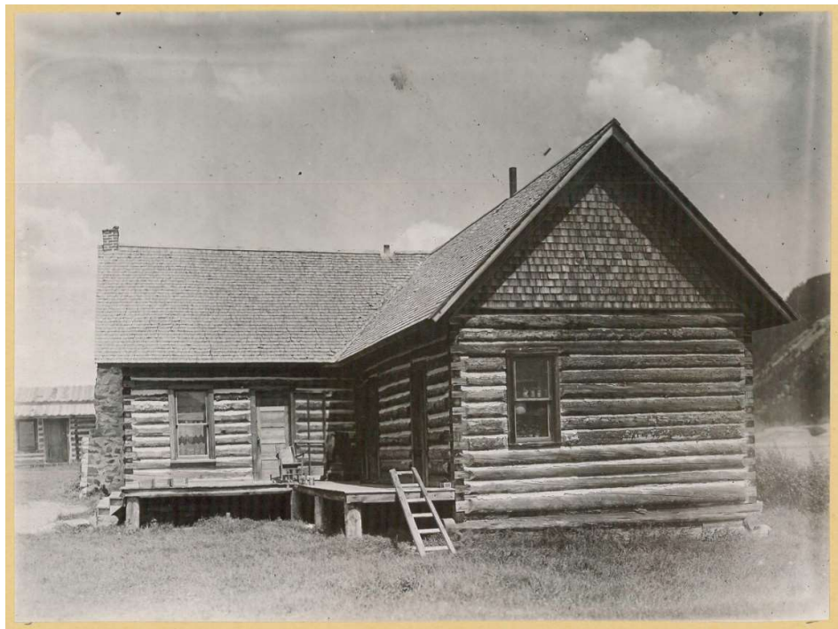
Fig.9. “Minidoka Project - Cottages near Jackson Lake Dam.” National Archives Catalog, catalog.archives.gov/id/100310733
