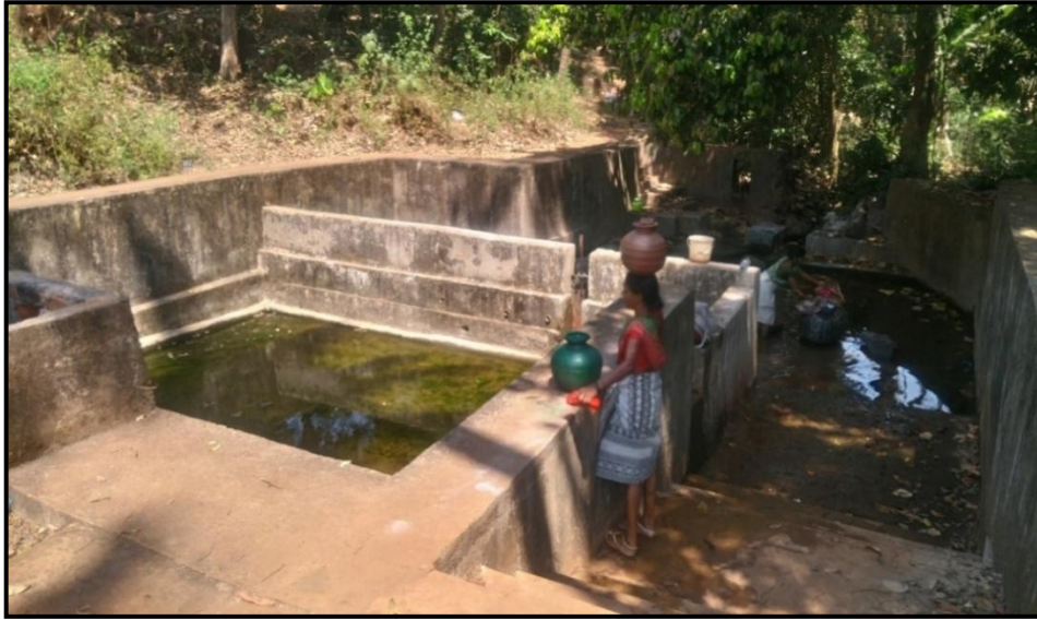
Figure.1.7: Water tank at Morlem
