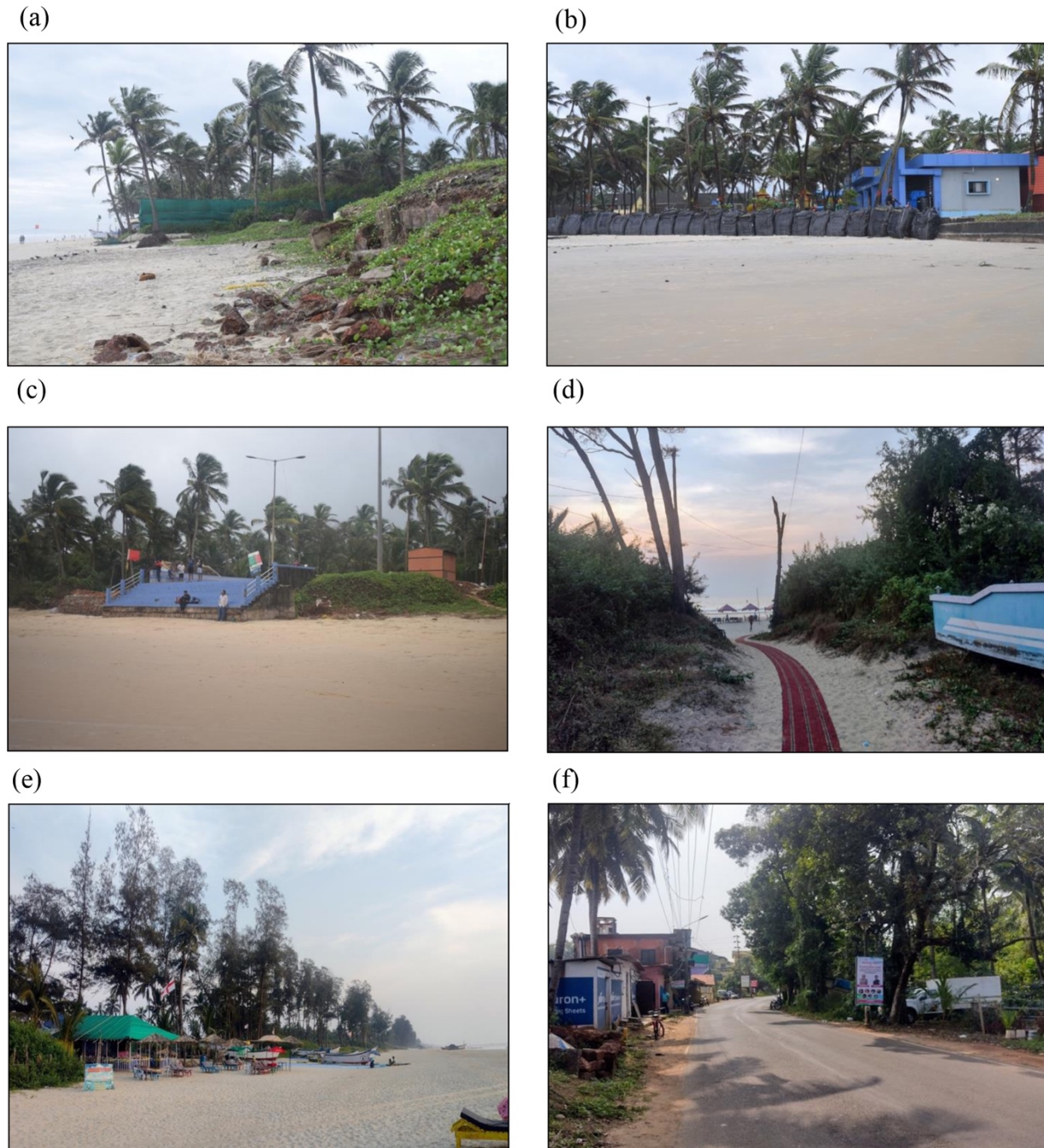
Fig –11.12 Status of sand dunes at various beaches in the study area. (a) Destroyed dunes at Colva beach, Salcete (b) Protection barriers (sand bags) to save infrastructure constructed on razed sand dunes, Colva beach, Salcete (c) Way to Velsao beach, Marmugao without razing stabilized sand dunes, (d) Way to Betalbatim beach, Marmugao constructed after razing stabilized sand dunes, (e) Protected vegetation (Casuarina plantation) and sand dunes with minimal tourist infrastructure at Gonsua beach, Salcete and (f) Showing limited connectivity, a Lone road connecting high-end tourist destinations of Cavellosim and Mobor villages, Salcete with the mainland.
