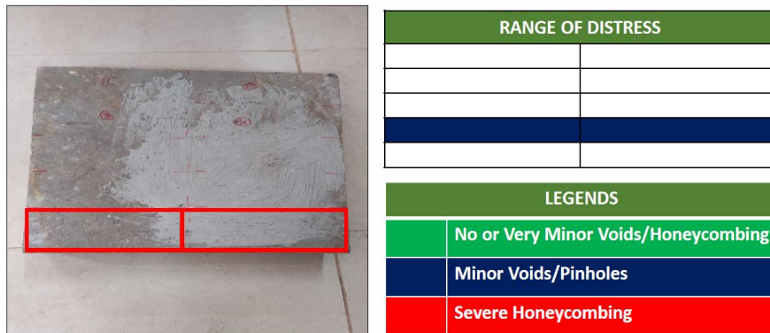
Figure 101 A-scan of surface. Red box shows the extent of area scanned.
