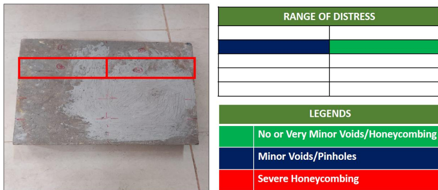
Figure 95 A-scan of surface. Red box shows the extent of area scanned.
