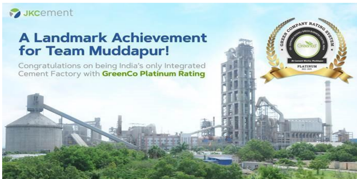
Figure 3.2: JKCL Plant at Muddapur, Karnataka accredited with GreenCo Platinum Rating
