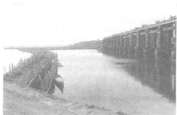
Enamavu regulator with a temporary 'mattom'.
